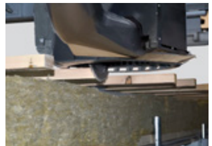
Formatting the roof battens
